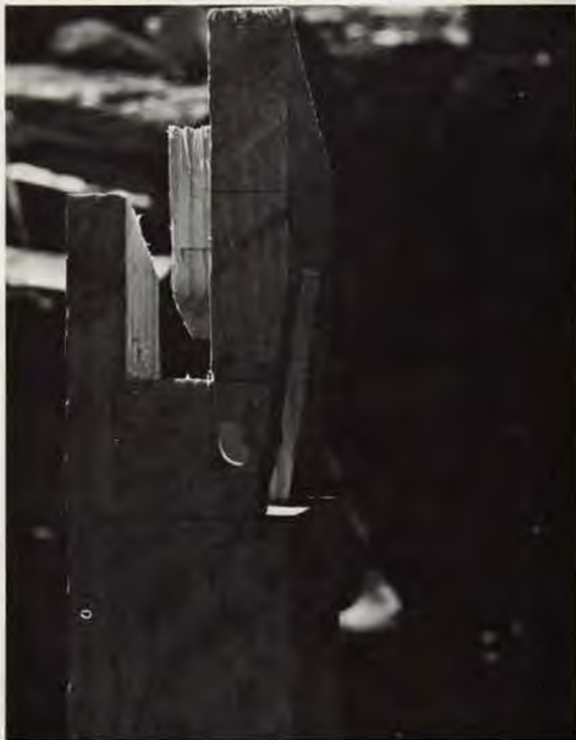
Compound hip post for the roof of the new kitchen
