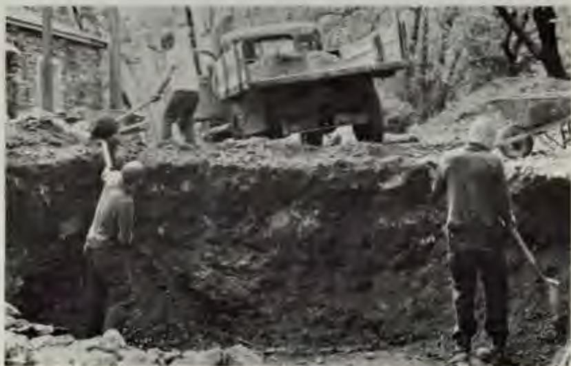
The leaching field hole
