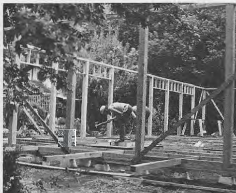
April 24: finishing the frame and installing the exterior walkway supports.
