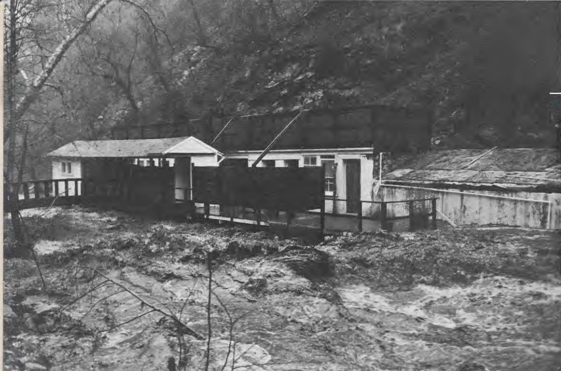
The bath bridge was later raised three feet to keep it from acting as a dam with branches and debris behind it.
