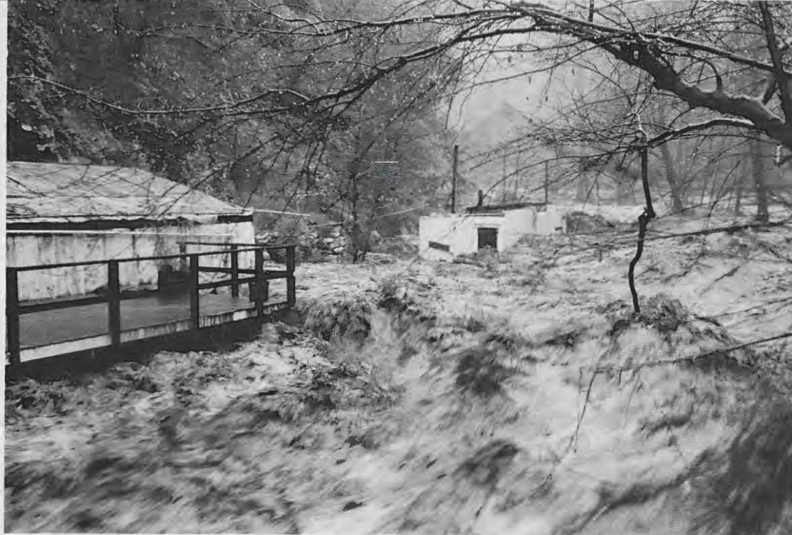
Soon after this photograph was taken the creek ran over the steam rooms (center) and up over the bath deck and into the hot-springs plunges.
