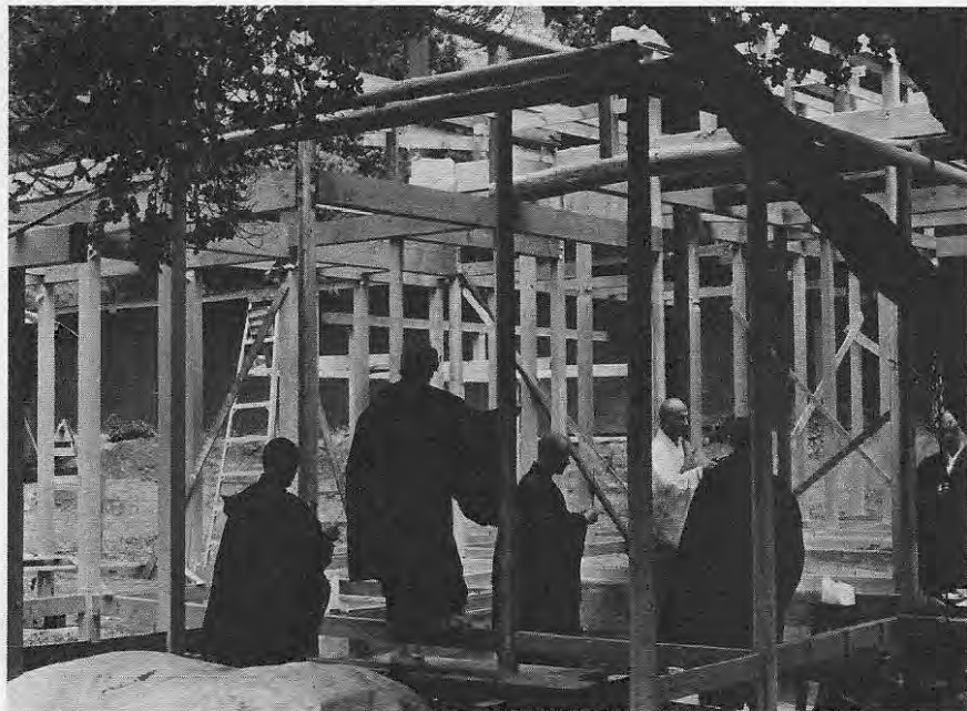
Dedication of the Teahouse at Green Gulch
