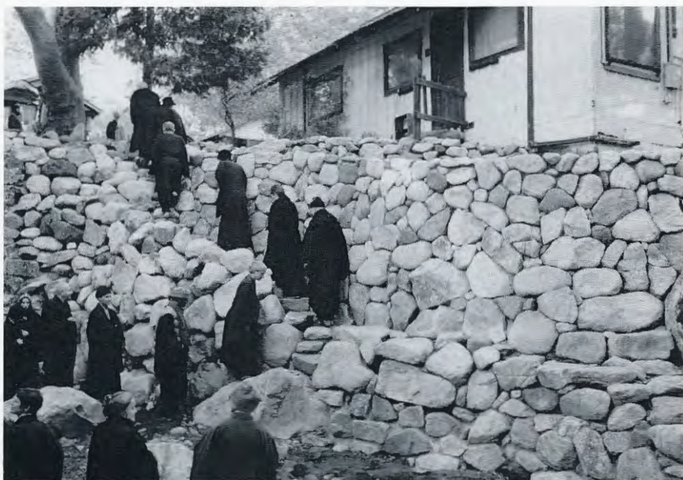
Ceremony at Tassajara to dedicate the new wall
