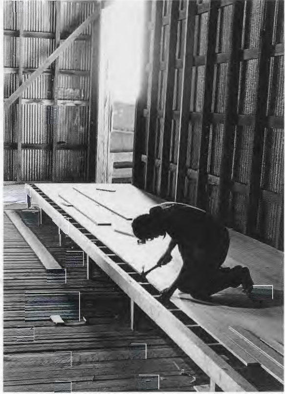
Building tans for zazen in the barn zendo
